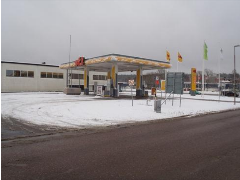
Foto 3: Fastighet Ladan 1, bensinstation.
